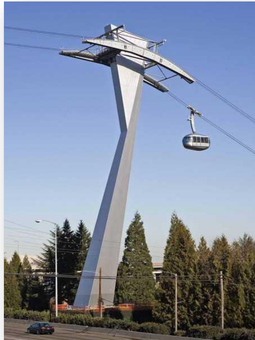
Figure 5: Portland Aerial Tram Tower
