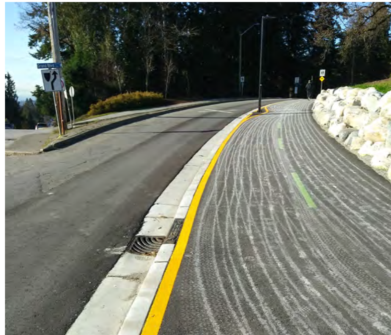
Signage and pavement markings on the Green Necklace Pathway in North Vancouver, B.C., showing shared pathway signage (top left), multi-use pathway pavement marking and green directional centre line striping (special colour used as pathway branding/wayfinding) (top right), hazard striping (bottom left) and edge line striping (bottom right).
