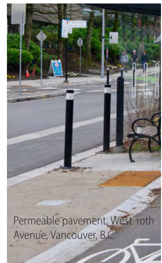
Exposed aggregate and unit pavers, Vancouver, B.C.
