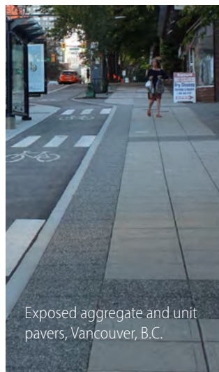
Permeable pavement, West 10th Avenue, Vancouver, B.C.
