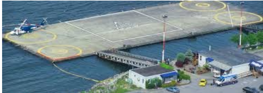
Figure 7 - Vancouver Harbour Heliport, a floating superstructure, can accommodate up to four parking positions and one FATO (final approach and takeoff) position for all category size helicopters. Shown is a Sikorsky S-76 parked. Main Passenger Terminal and Cargo Terminal are situated on the shoreline. Scheduled service operations to Victoria and other destinations can be booked daily from this public heliport facility.
